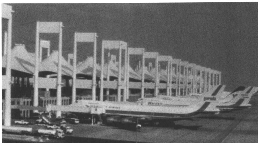
Figure 6. Fabric roof of Saudi Arabian Airport Terminal: (a) inside and (b) outside
