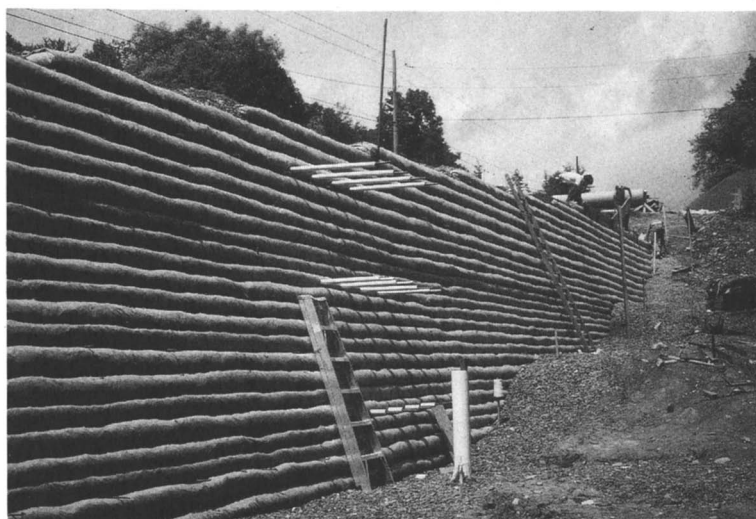
Figure 4. Reinforcement (wall) application.
