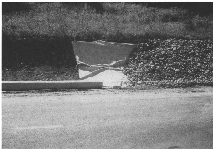
Figure 6. Slope protection application.
