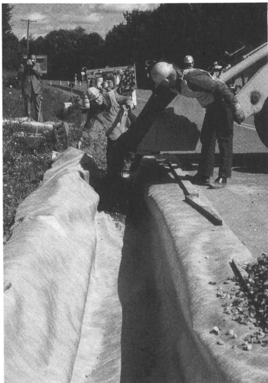
Figure 3. Underdrain (drainage) application.
